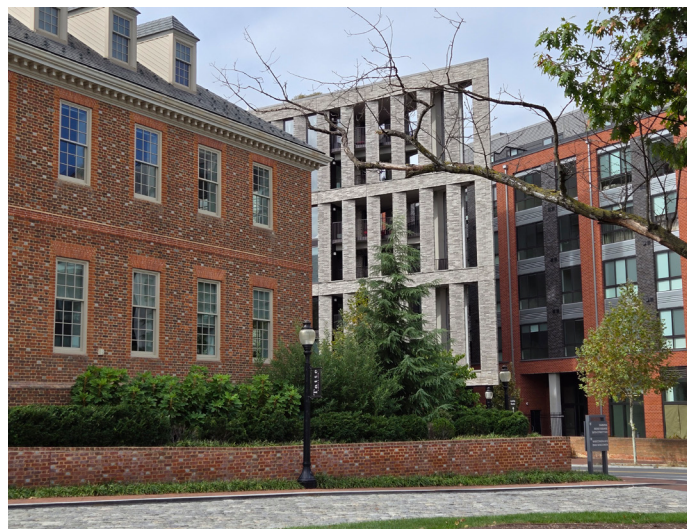
Photo 2: Existing building with brick structural walls (left) renovated and reused within new development
