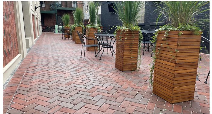
Photo 1: Permeable clay brick pavement
